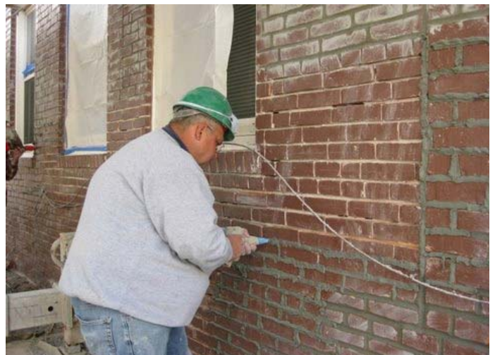
Ron O'Neil tuckpointing, like a dentist filling cavities
